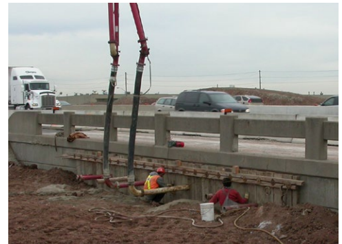
CBM's FlowFill is best suited to areas that safety or physical constraints hamper compaction.
