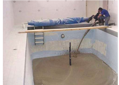
CBM's FlowFill is best suited to areas that safety or physical constraints hamper compaction.
